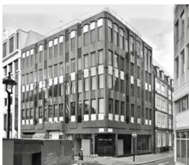
The existing Dacre House
