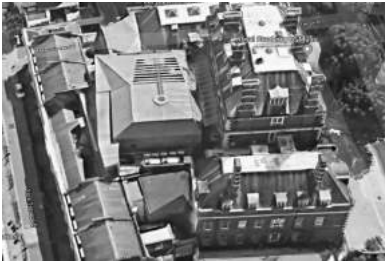
The Royal College of Music site with the stuffed-in addition embracing its new spaces
