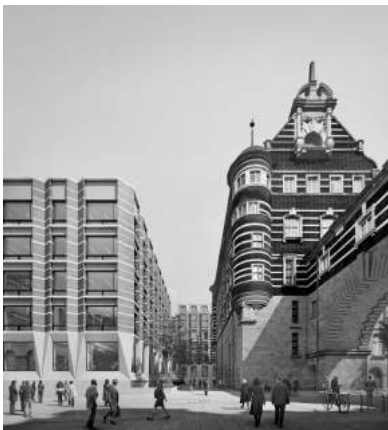
New façade elements for the Northern Estate. Existing Norman Shaw building to the right
