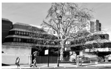
Two present views of Belgravia Police Station
