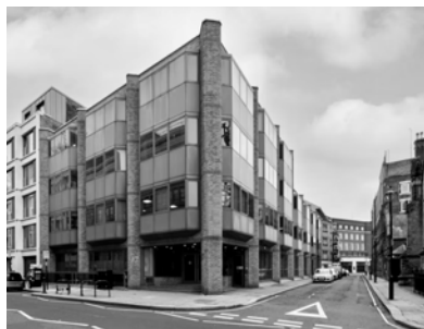
Rochester Row's orange brickwork and metal panels
